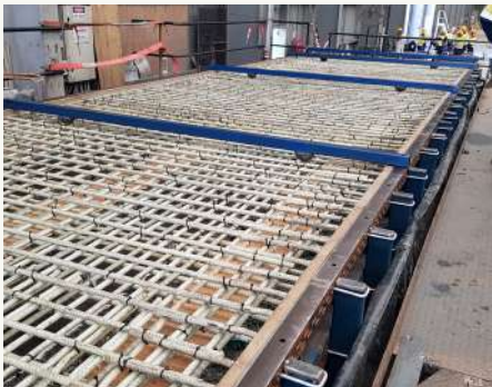
REINFORCING FRP REBAR
