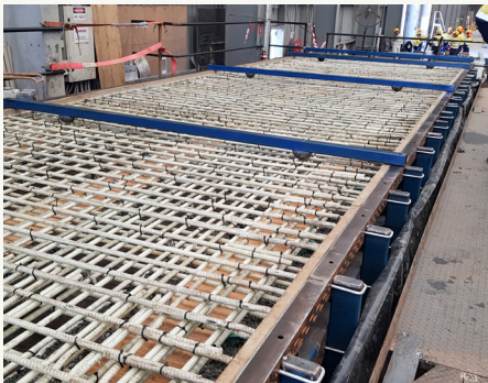
REINFORCING FRP REBAR
